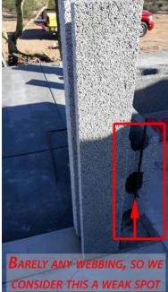
This photo shows the block wall prior to grouting and prior to scraping the tack glue from the face of the wall. Notice the "fish plating" where we have identified areas of concern. The minimal exterior bracing is also a precaution. The top corner of the wall is blocking for a beam seat.
