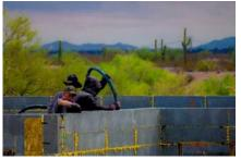
**Builder's Tip:** Before grouting, having a visible spray paint mark on the face of the wall at the top for proper placement of anchor bolts. This technique can save costly omission and placement mistakes. An anchor bolt must be placed within 12" of the end of each length of top plate board. Consider whether you will have butt or miter joints for your top plate boards at each of the corners and the length of the boards you will use and place your paint marks accordingly.
